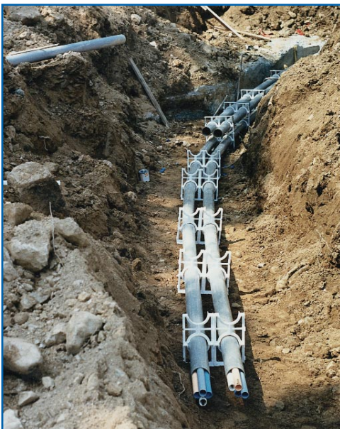
Pulled through existing conduits
