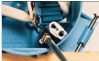
Pre-installed Lugs
