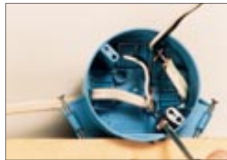
Make Grounding Connection
