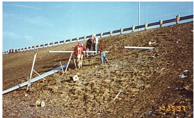
Above: Bore-Gard PVC pipe is being installed on a 45 degree slope near the intersection of Ohio Interstate 271 and Route 480 near Cleveland. Two 220 ft. installations were made about 20 feet apart under the active highway. In spite of the challenging terrain, the pipes were easily assembled and locked together before being installed.
