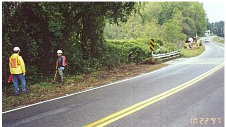
Left: Facing the drilling rig (top left) overlooking the creek. Directional drilling and Bore-Gard pipe was the least cost option for this varied-terrain 180 ft. bore. Trenching was not an option. Above Right: A look at the 180 ft. span of the bore from far left to far right (drill rig) of the picture.
