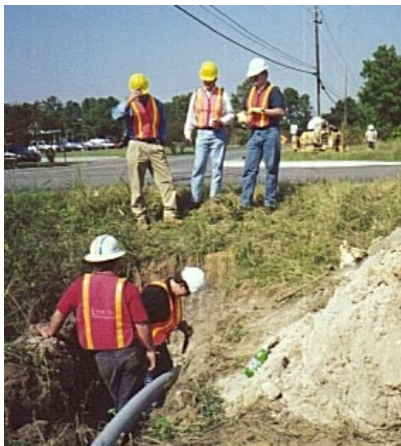
Above Left: Bore-Gard PVC pipe at a depth of 6 feet is being pulled beneath the active roadway. The tight transition and resultant bend radius was no problem for the strong joint design. Above Right: The entire Telco company crew was impressed with the simplicity, fast assembly, and strength of Bore-Gard. The entire 100 feet of pipe was laid out in a few minutes for before the installation.
