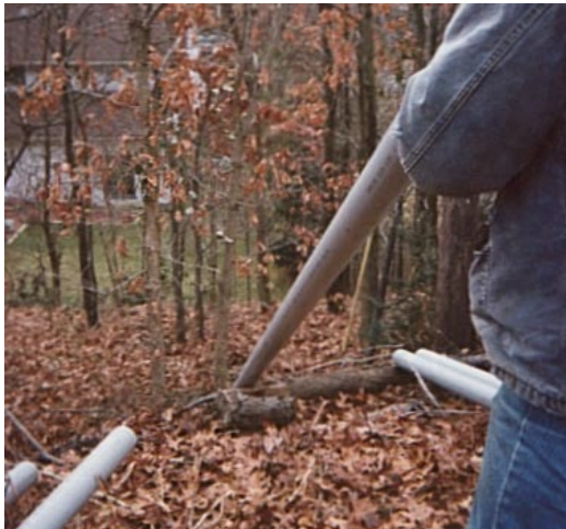
Above Left: Bore-Gard PVC pipe being installed down a 45 degree slope behind a residence. The elevation change was 50 feet from the residence yard below. Above Right: View from the drill rig. The bore path went under the street, beside the residence and up the hill behind the home - a total of 220 ft.
