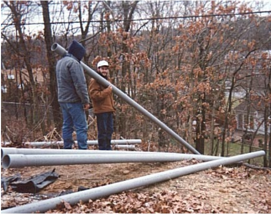
Above Left: Bore-Gard PVC pipe being installed down a 45 degree slope behind a residence. The elevation change was 50 feet from the residence yard below. Above Right: View from the drill rig. The bore path went under the street, beside the residence and up the hill behind the home - a total of 220 ft.
