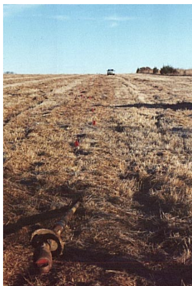
Above Left: Bore-Gard PVC pipe is being attached to the Condux ® pulling eye and Ditch Witch ® 8 inch "Beaver Tail" reamer. Above Right: Bore-Gard pipe before the 1,000 ft. installation.
