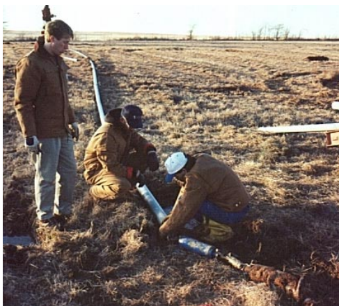
Above Left: Bore-Gard PVC pipe is being attached to the Condux ® pulling eye and Ditch Witch ® 8 inch "Beaver Tail" reamer. Above Right: Bore-Gard pipe before the 1,000 ft. installation.
