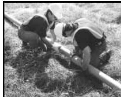
Attach the next piece of Bore-Gard.
